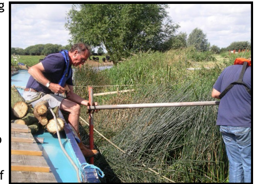
Ernest Boddy placing fittings to the temporary moorings
