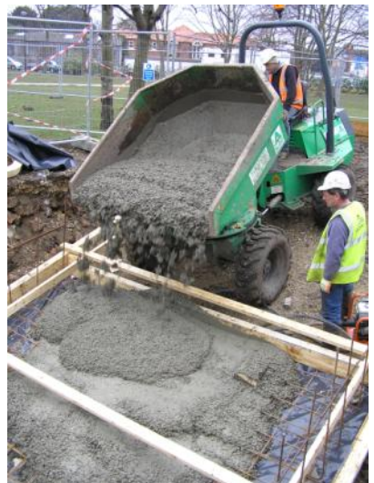
Concreting the slipway
