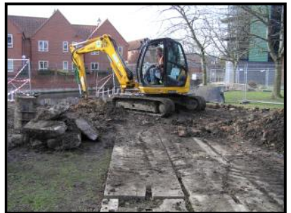
The “Bogmat” tree protection system in use
