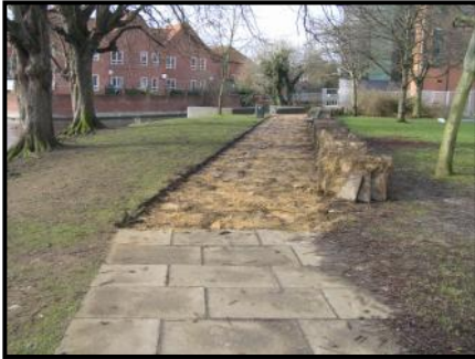
Removal of old path
