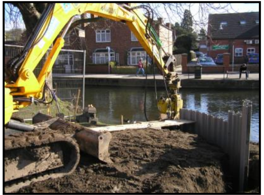
The piling system, and piling in progress
