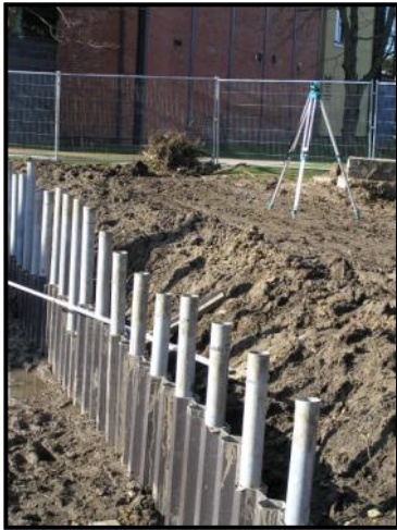
The piling system, and piling in progress
